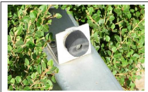
Ensure stops are installed on the gate for the fully closed and fully open positions.
