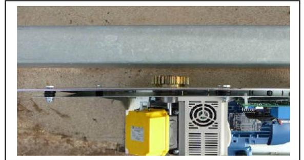
Fix rack to the gate frame keeping 1mm-2mm clearance between the rack teeth and Pinion wheel
