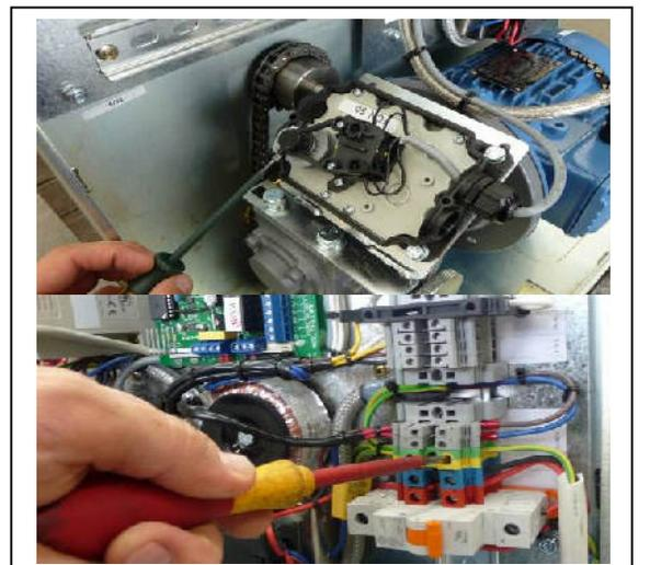
To commission the gate, move the gate approximately 1m from the fully open position and tighten the knurled wheel (Clockwise) engaging the clutch assembly
