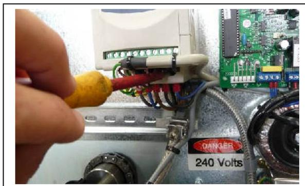
**Ensure** the direction the gate travels is in accordance with the opening and closing status LED's, if not reverse two of the motor wires at the inverter terminals.
